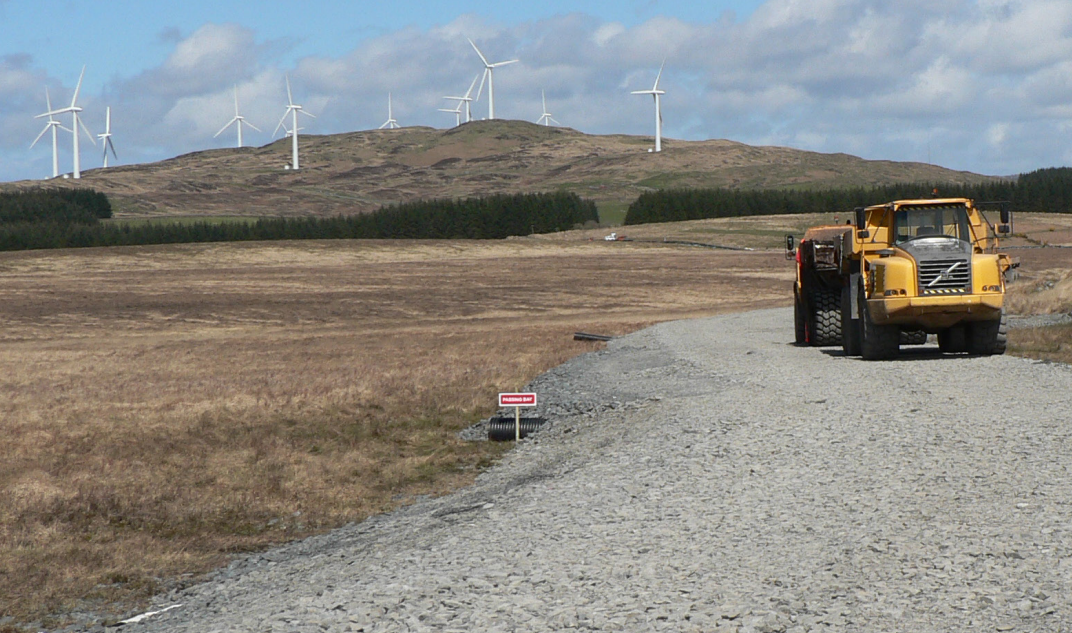
The access road crossed over an area of very soft peat bog.
