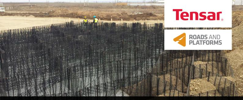
The TensarTech Stratum Cellular Foundation Mattress was assembled on site by hand, enabling it to be built quickly and easily on the soft ground, in all weathers.
